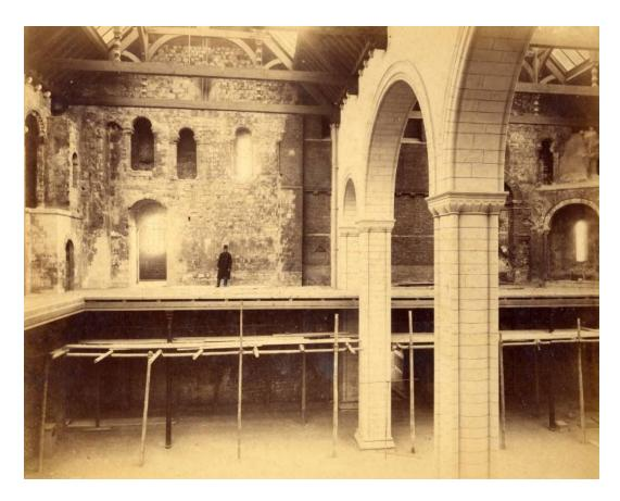
Modern arches, designed to look Norman like the Keep, were inserted to hold up the new roof, and a wooden walkway inserted around the edge
