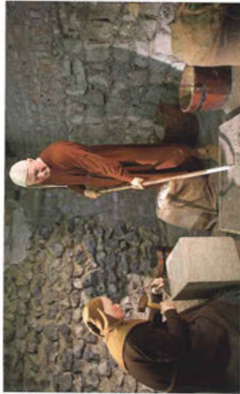
ABOVE A mason dressing or cutting stone whilst an assistant mixes mortar in a mortar pit
